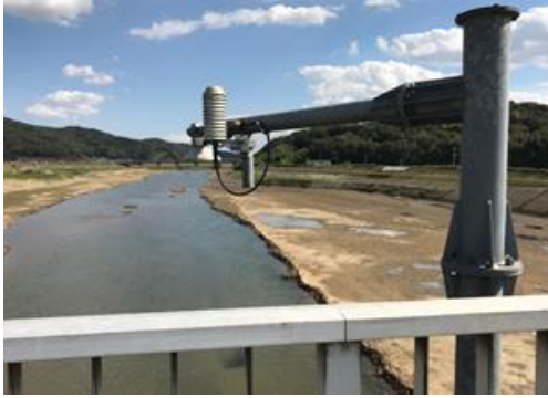
Fig. 7 The water level observation in Yakatabashi The first author took the picture on October 29, 2018.
