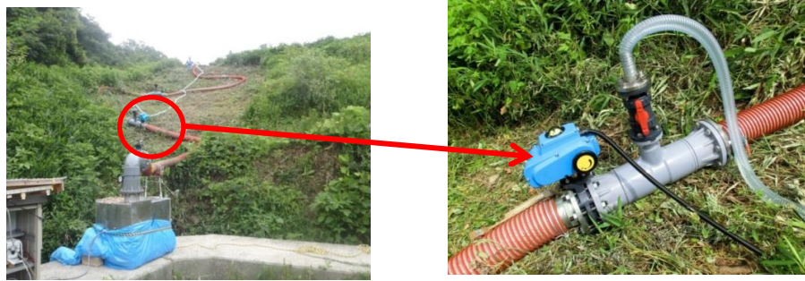
Pic. 1 Installation of an electric bulb (Left: outlines of hydroelectric system)
