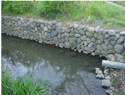
Fig. 1 Example of (a) masonry and (b) wooden revetment works in canals Riparian plants grow between the wooden stakes
