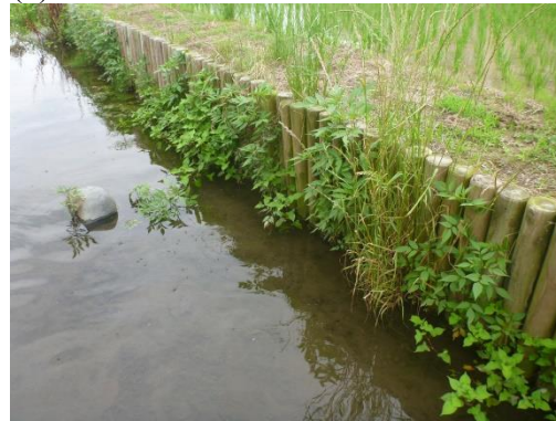
Fig. 1 Example of (a) masonry and (b) wooden revetment works in canals Riparian plants grow between the wooden stakes
