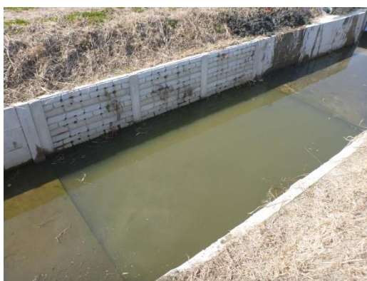
Fig. 4 Example of a habitat pool installed in a drainage canal
