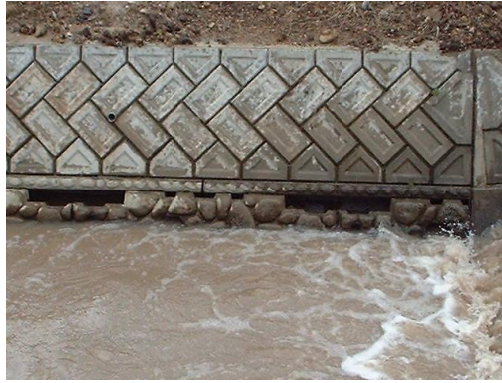
Fig. 2 Example of a concrete block habitat installed in a drainage canal
