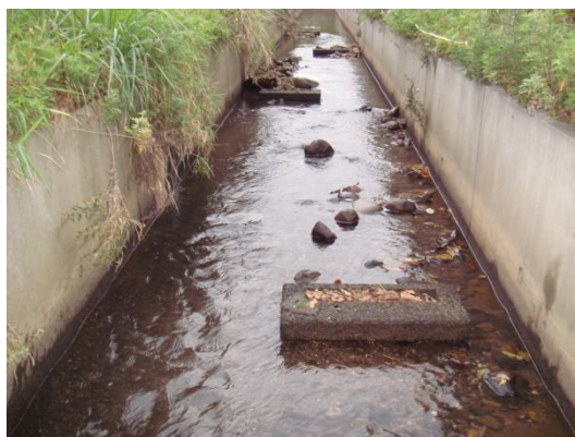
Fig. 5 Example of concrete blocks on the concrete lined canal bed
