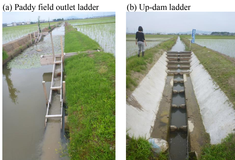
Fig. 7 Example of the two type of fish ladders in use
