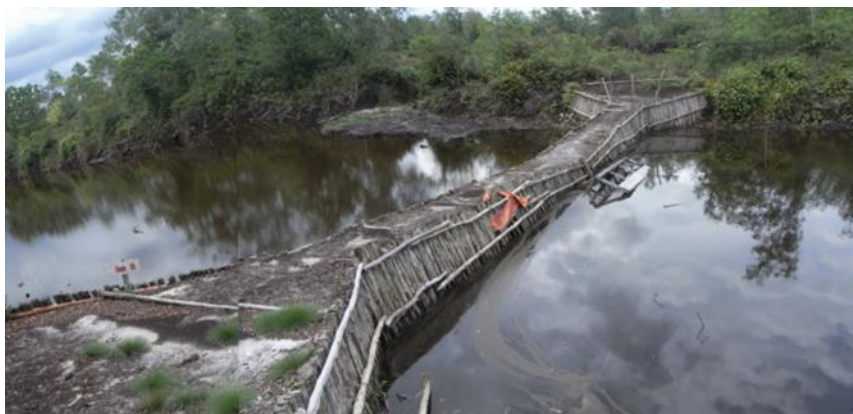
Fig. 1 Dam constructed in the canal near the restored forest
