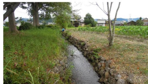
d) Irrigation Canal B
