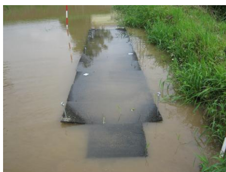
Fig. 3 Artificial floating islands wired each other and placed on biotope surface
